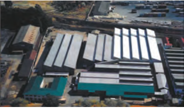
Germiston Head Office, Sales, Despatch & Factory
